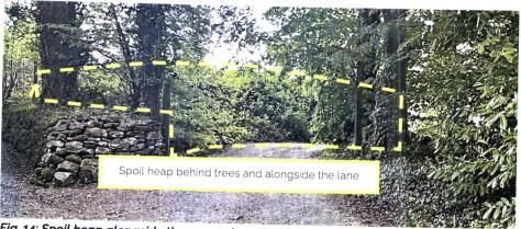
Fig. 14: Spoil heap alongside the access lane to clients' property
