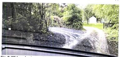
Fig. 8: Widened entrance & spread hard core stone replaces overgrown access
